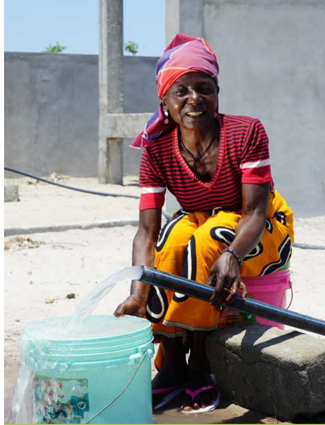
Molia Abdallah, 47, fills a bucket of water at the solar-powered water scheme being constructed in Chicoma, Nampula Province, Mozambique.
